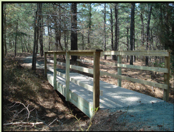
Typical Trail Bridge
