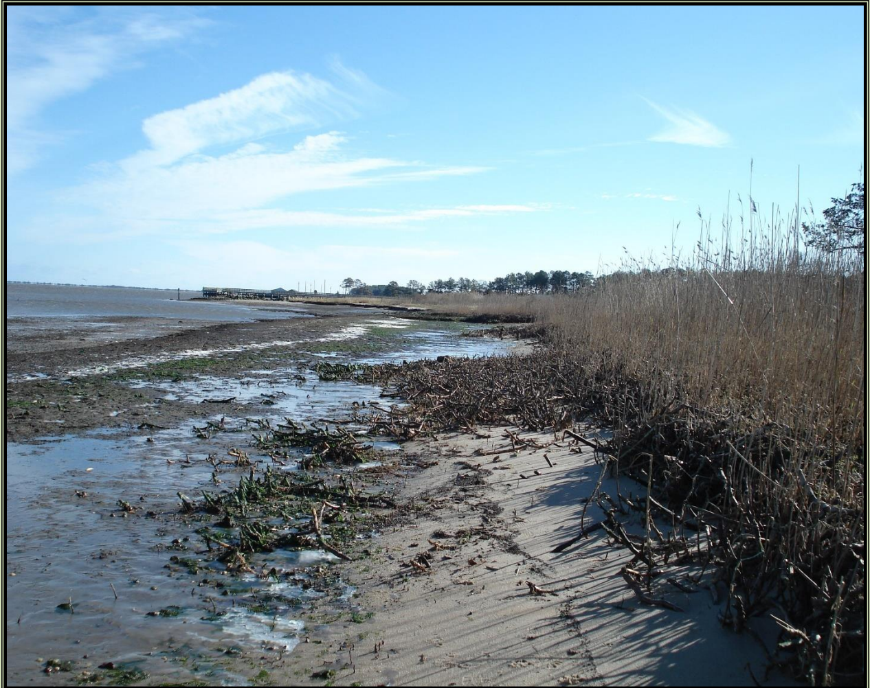
Indian River Bay Shoreline Erosion – fall 2009 (View to the east)
