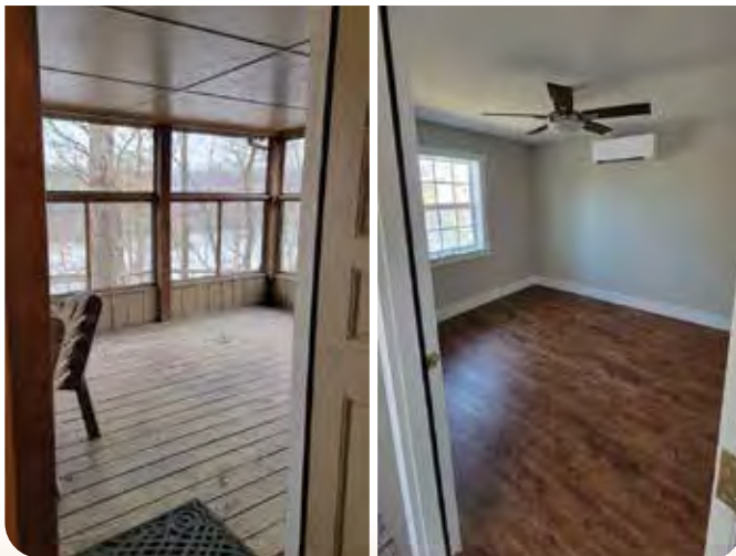
Killens Pond State Park Pond View Cottage conversion of porch to additional bedroom
