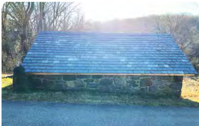
Rebuilt roof at Spring House in Brandywine Creek State Park
