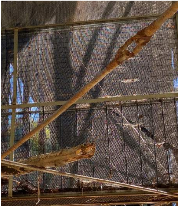
Corroded Tie Rod and Coupler
